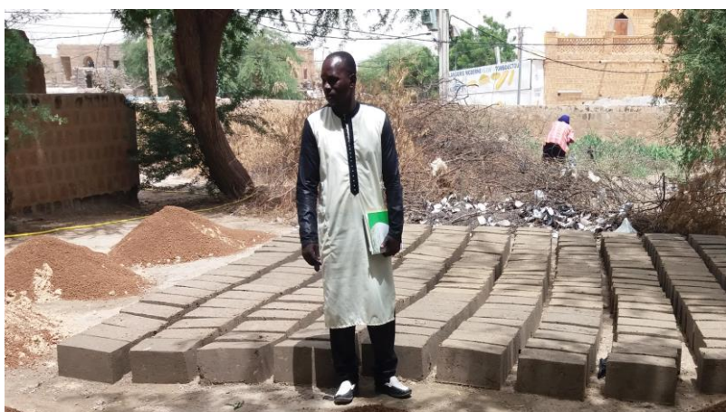
Making bricks to start on the new toilets
